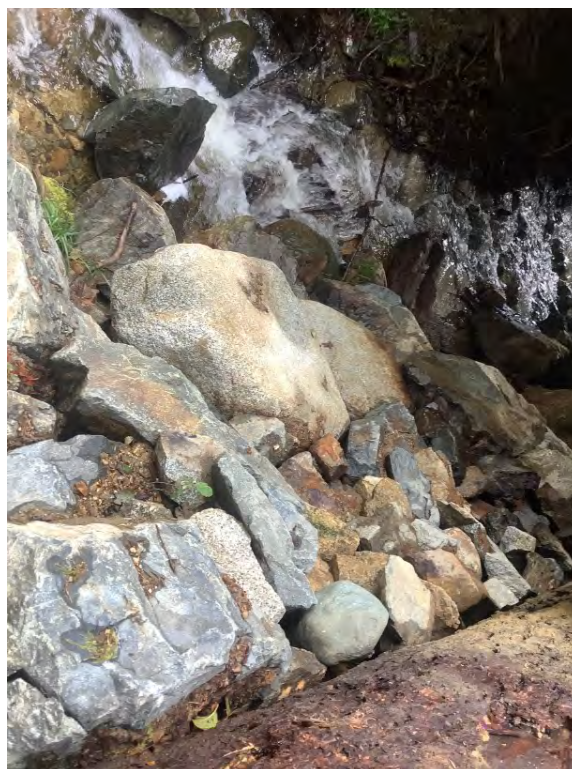
Left Bank Abutment when facing downstream
