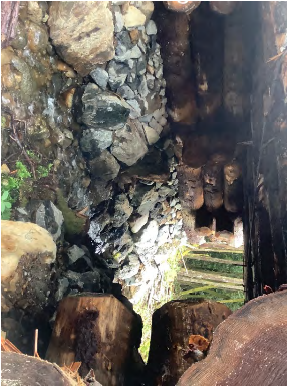
Left Bank Abutment when facing downstream
