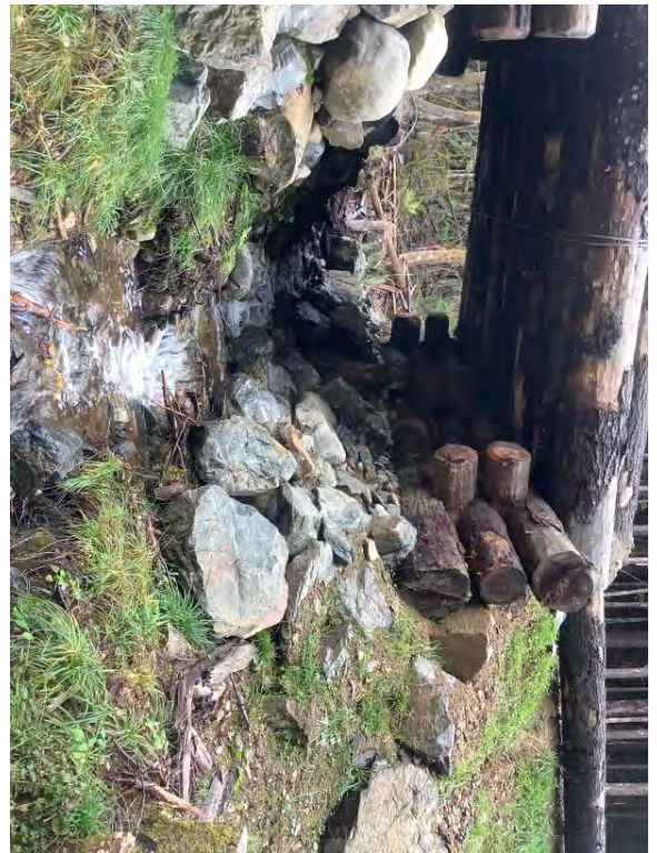
Left Bank Abutment when facing downstream
