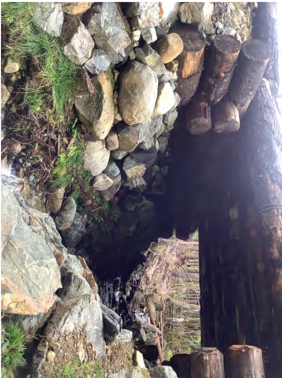
Right Bank Abutment when facing downstream
