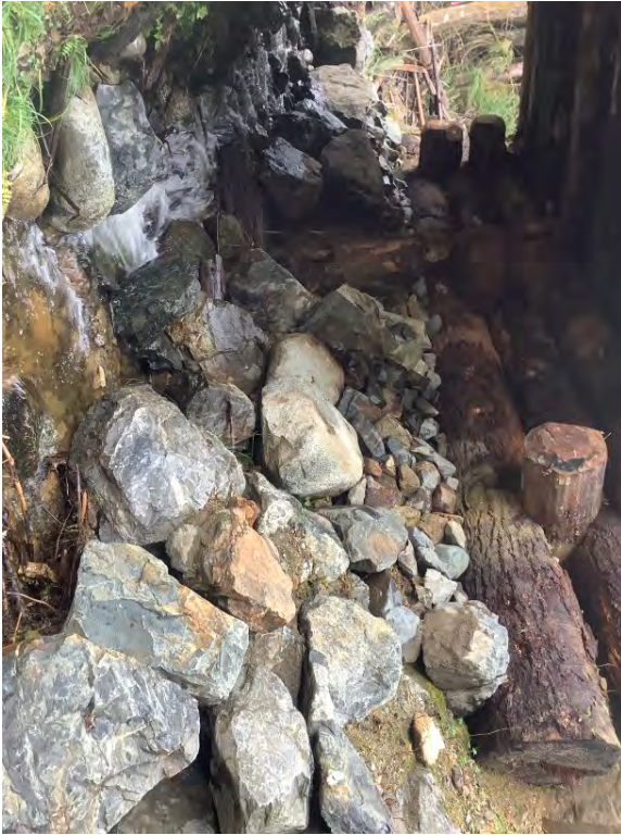
Left Bank Abutment when facing downstream
